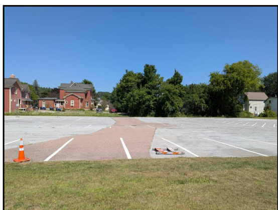
5: View from the middle of the Subject Property looking north. Drain #3 in middle of pavement patch
